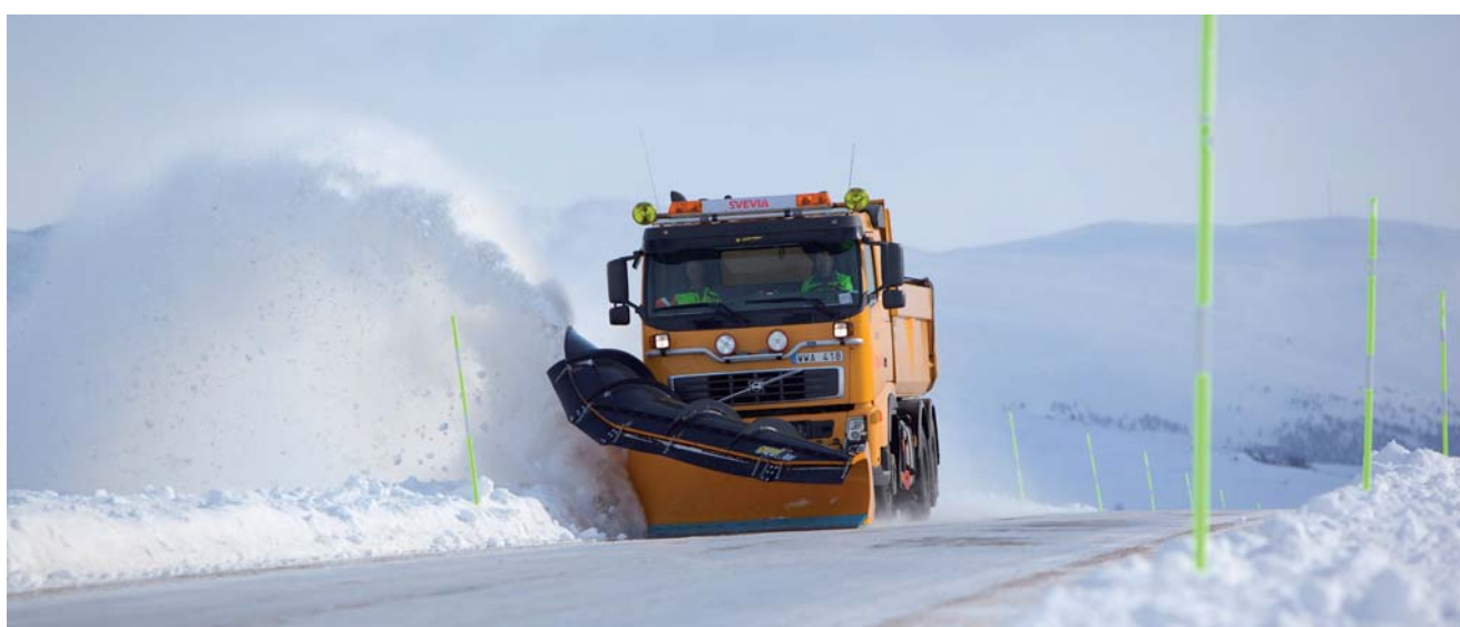
In the operation and maintenance of roads, Svevia is the market leader in Sweden with a market share of slightly less than 30 per cent the country's road network. Photo: Patrick Trägårdh/Svevia
