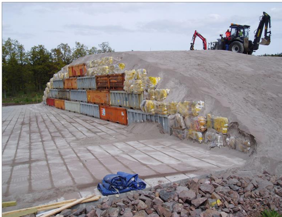
Figure D5 The shallow landfill facility at OKG
