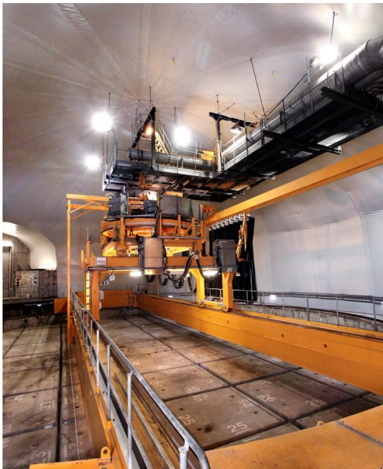
Figure A8 Photo from the top of the silo in SFR
