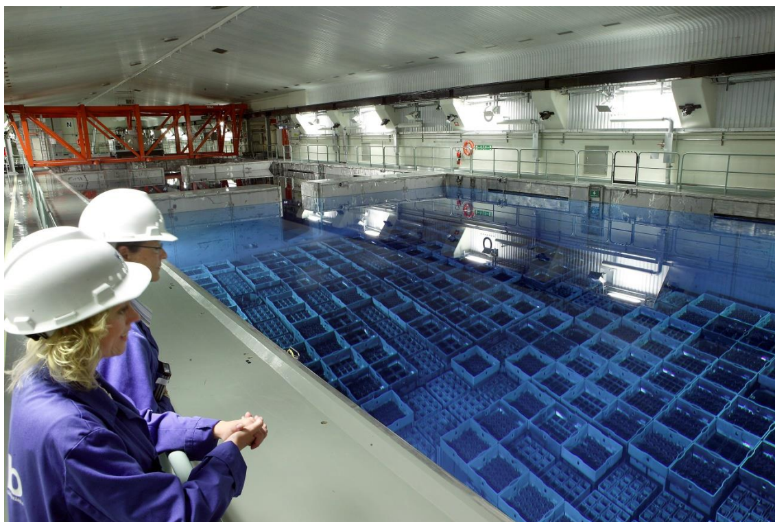
Figure A5 Storage pool in Clab
