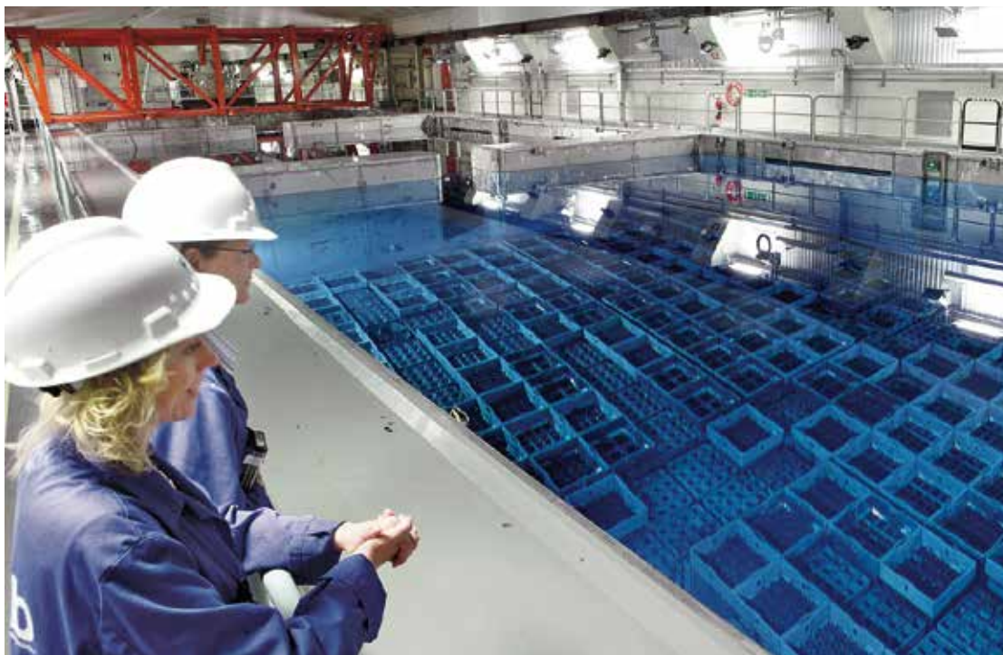
Figure A6: Storage pool in Clab.
