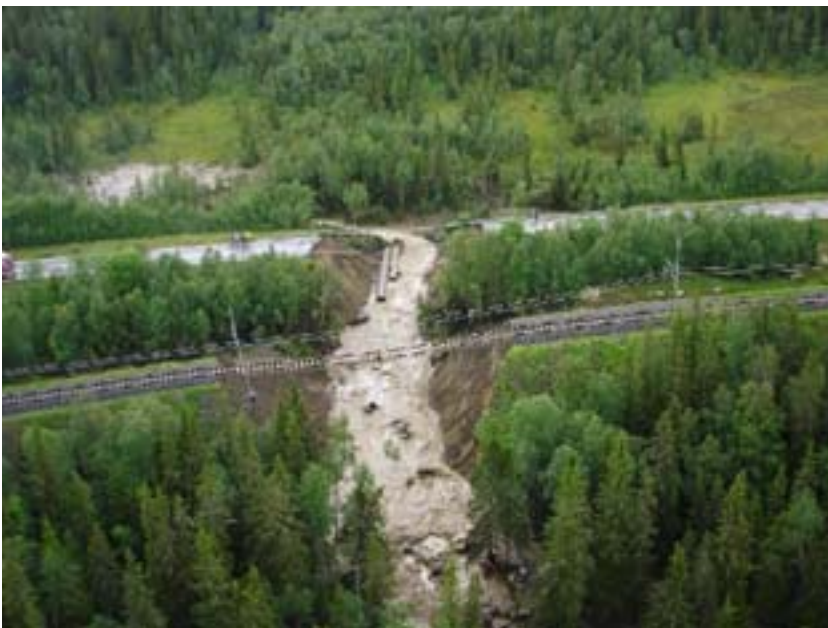
Picture 3.1 The rockslide in Ånn in summer 2006
