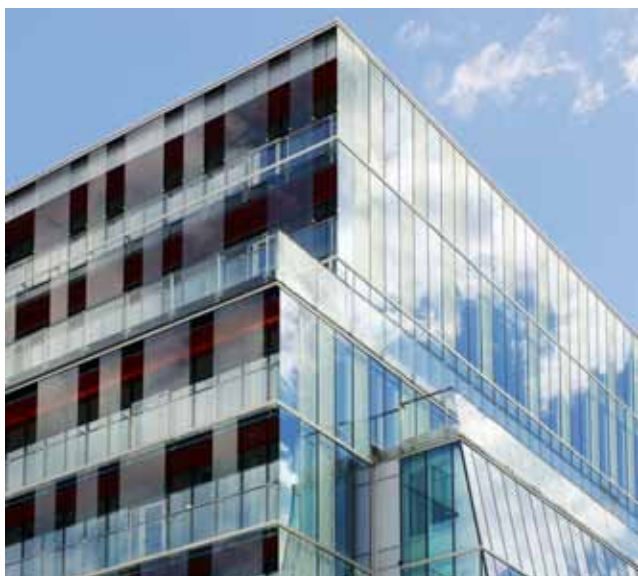
Jernhusen's newly-built and climate-smart building Kungsbrohuset in Stockholm is proof that environmental investments pay off. Photo: Åke E:son Lindman/Jernhusen
