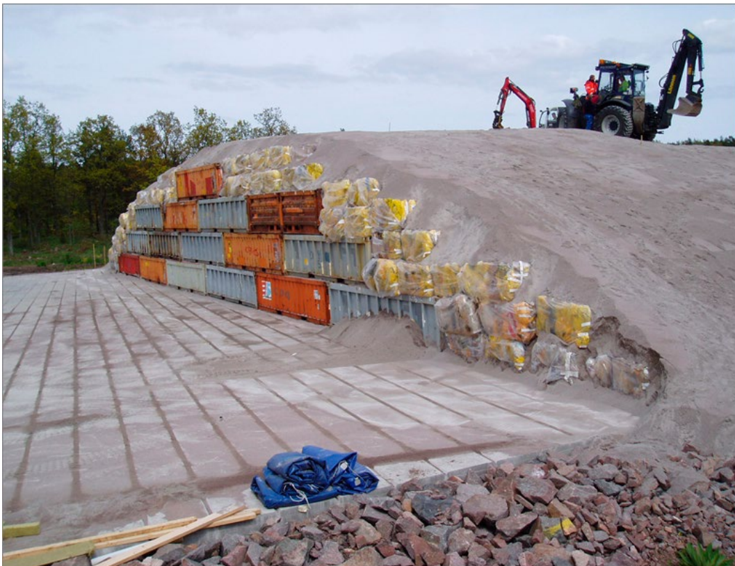
Figure D6 The shallow land burial at OKG.
