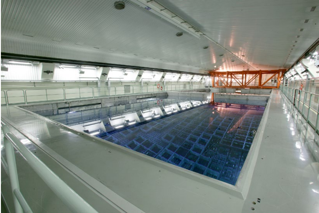
Figure A7 Storage pool in Clab. The top edge of the spent fuel is 8 m below the water surface.
