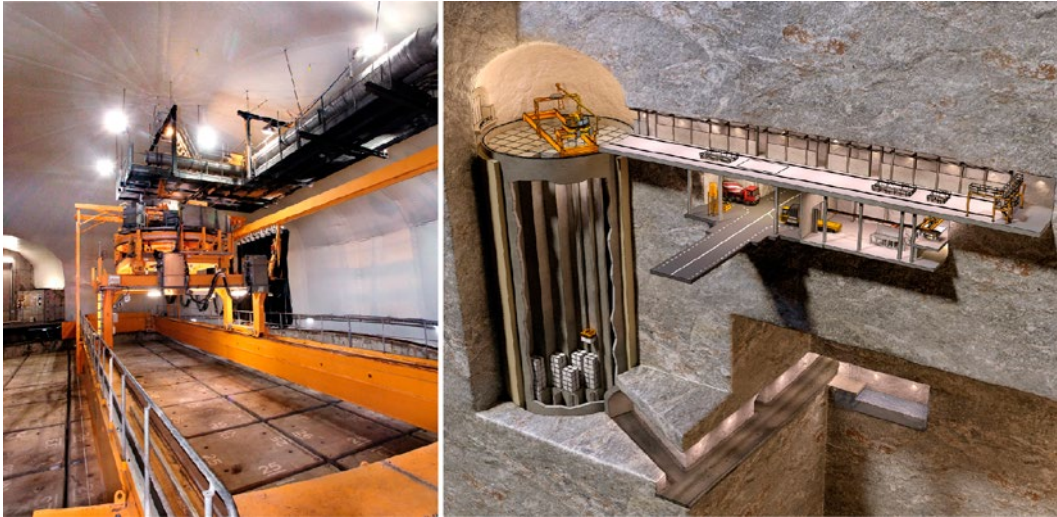
Figure A12 Photo from the top of the silo in SFR and an illustration of the design. Waste packages are placed in shafts in the silo.
