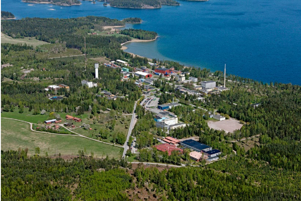
Figure A10 The facilities at Studsvik Tech Park.
